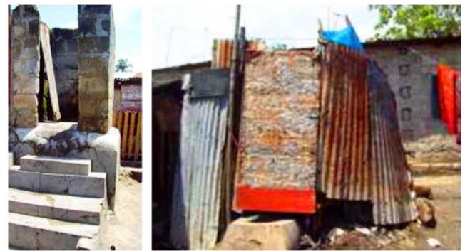
Figure 5.12. The lack of privacy in “passport size” unroofed toilet, as displayed on the (Left), unroofed toilet (“passport size”) raised built by block walls with foundation, and (Right)unroofed toilet (“passport size”) built by using corrugated iron sheet within Mlalakuwa area, Source: Authors, (2023)
