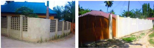
Figure 5.9. (Left) louvered block wall to enhance visual privacy, (Right) block wall as high up to 3m within Mlalakuwa area, Source: Authors, (2023)
