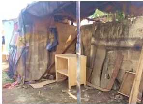
Plate 4.25: a woodwork or timber workshop improvised on urban space, in Sinza "A", Source: Author, (2024).
