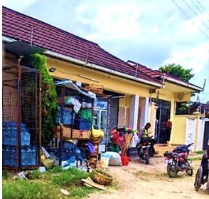
Plate 4.13: a retail shop, with improvised cages housing retail products, female boutiques, and motorcycle operators (bodaboda), in Sinza "A", Source: Author, (2024).
