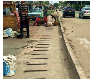
Plate 4.04: a piled up collected solid waste awaiting routine weekly LGA collection truck while blocking the pedestrian walkway along Mori Road in Sinza “A”, Source: Author, (2024).
