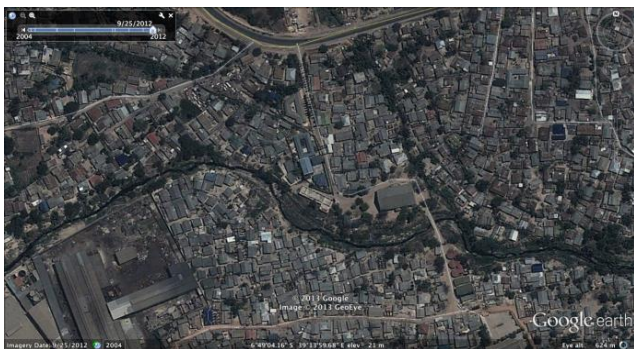
Image 3.3. Uncontrolled surface runoff from unplanned neighborhood flows toward the site. Source: Adapted from (Google Map, 2025)
