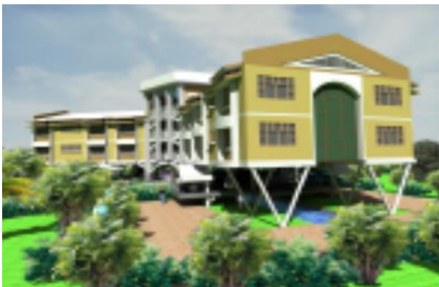
Image 6.16. Shows the safe zones/building with suspended piles for flood precautions. Source: Field survey, (2025)
