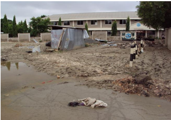
Image 3.7. Flood impacts on MEMKWA premises. Source: Field survey (2025)
