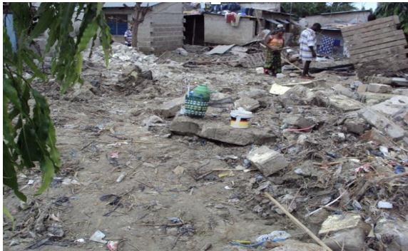
Image 3.6. Flood damage observed beside Luhanga Catholic Church quaters. Source: Field survey (2025)
