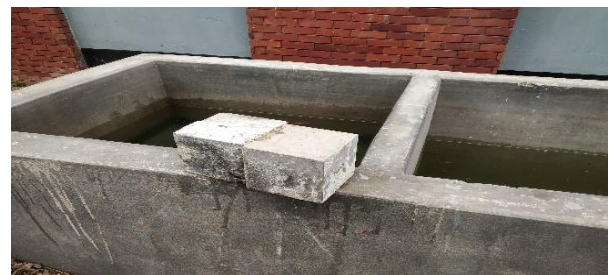
Figure 10. Efflorescence
