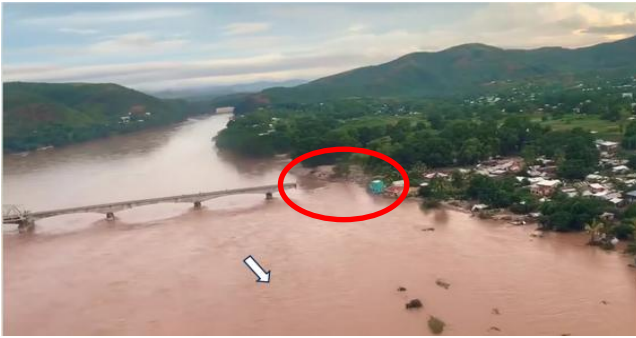
Figure 1. View of the bridge over the Mahavavy river and the partially destroyed section
