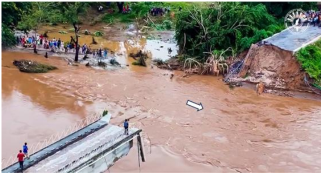
Figure 2. The left-bank abutment and part of the bridge were swept away by the flooding of the Mahavavy river
