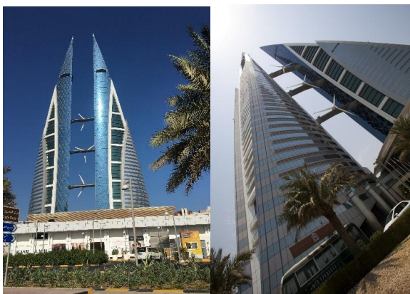
Figure 8. Bahrain WTC the first skyscraper in the world to integrate wind turbines into its design. Source ( http://www.skyscrapercenter.com )
