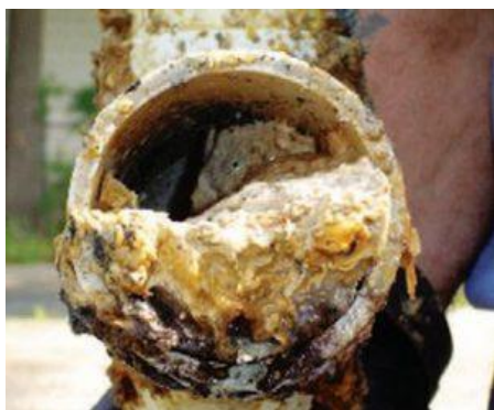
Figure 3. FOG Residue Clogging Local Drains Connected to Sewers (Source: Unknown (2021)) [24])
