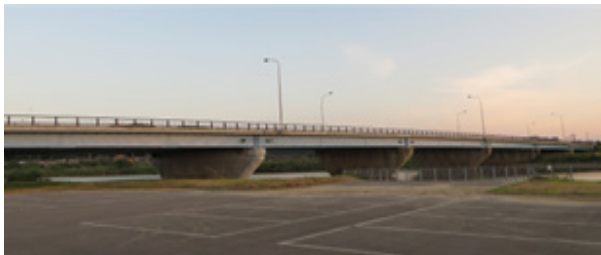
Figure 2. Target bridge for measurements (Asuka Ohashi Bridge). The bridge comprises seven spans having total length of 256 m. Experimental measurements were taken of the first span near the left abutment
