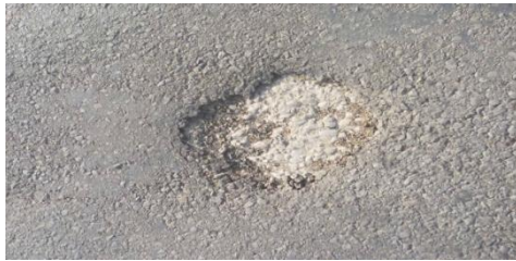
Figure 1. Potholes
