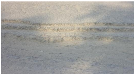
Figure 3. Edge cracking
