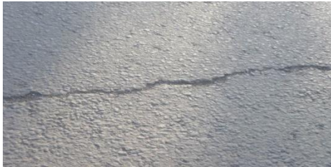
Figure 2. Longitudinal cracking
