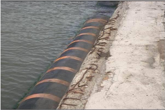
Figure 4. Corroded steel reinforcement bars at quay edge beam
