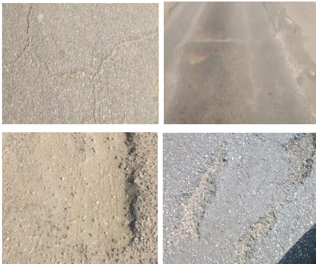
Figure 2. Asphalt concrete pavement distress
