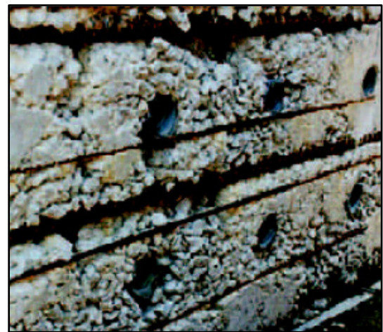
Figure 4. Cracking due to corrosion [11]
